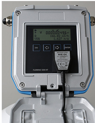
Fig. 40 Aligning the infrared/USB adapter
