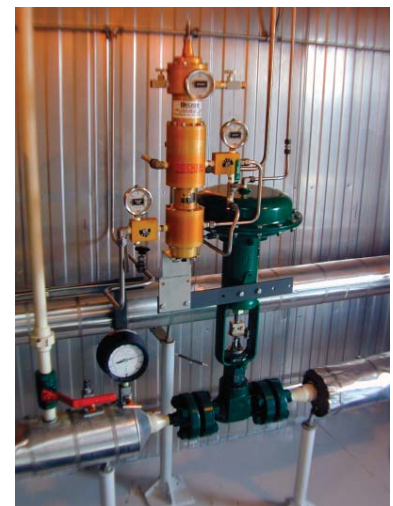
Figure 8 - VRP-SB-CH Retrofit Virtually Eliminates Atmospheric Bleed Gas
