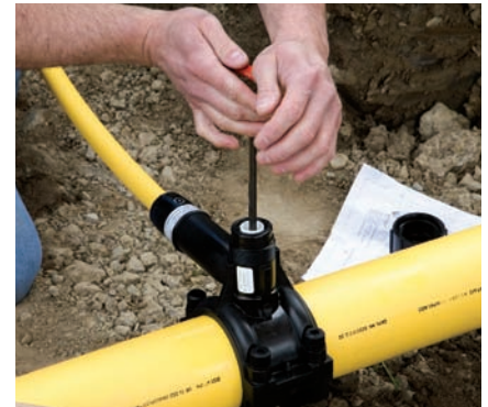
By-pass is made easy with a PermaLock tapping tee
